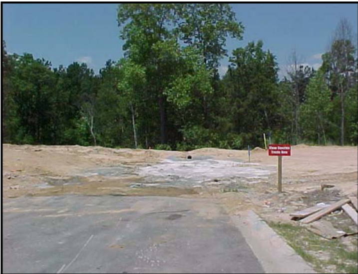
Looking at site from Grandview Cir.
