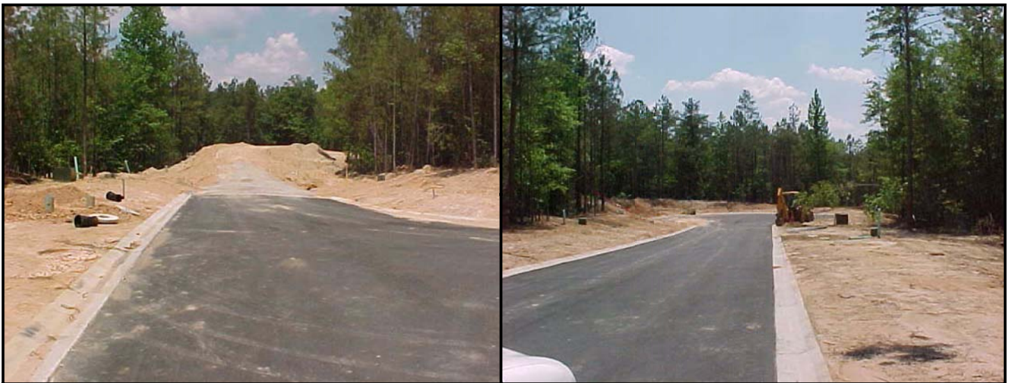
Looking at site from Berkeley Ridge Dr.
